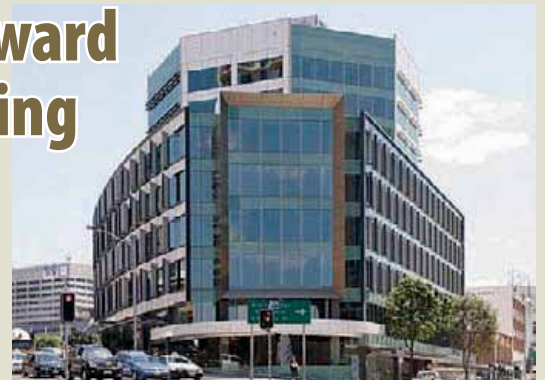
The construction site on a virtual traffic island was a major challenge for Hutchies' team at 545 Queen St.
