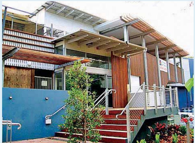
HUTCHIES' Noosa office has completed the Noosa Surf Club refurbishment and extensions and the new Noosa Visitor Centre, built as separate contracts on adjoining sites.
