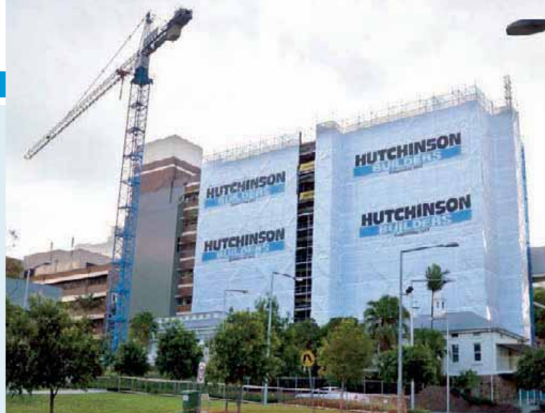
University of Queensland, Health Sciences Building. Job value $21.6M.
